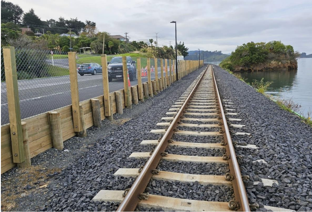
Figure 18. Timber retaining wall and fence between trail and railway line.
