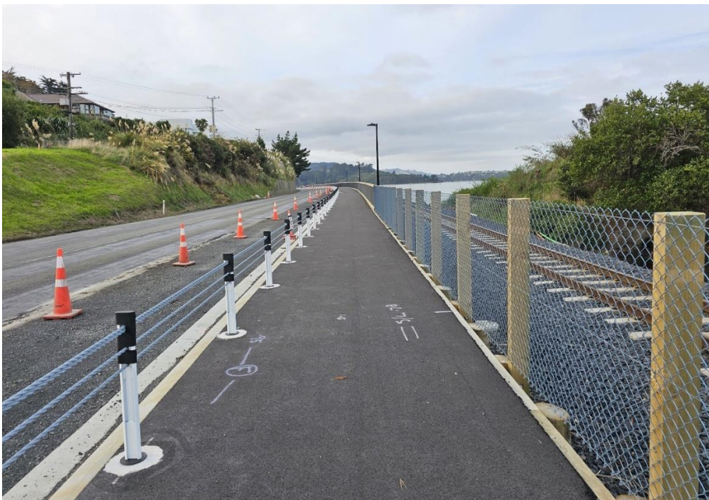
Figure 19. Wire rope barrier between trail and highway.
